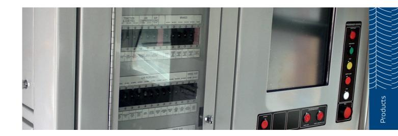
Available technologies include a wide range of Bus Interface Modules (e.g. WTB, MVB, CAN, Serial Links and Ethernet) and Input/ Output Interface Modules (Analogue Input, High Speed Analogue Input, Digital Input/Output, Digital Relay Output, Analogue Output, Pt-100 temperature Sensor Input). Remote Input/Output Modules (RIOM) are also available.
